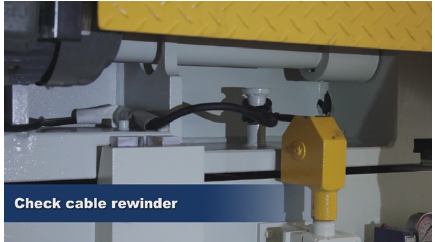
Bolster cable problem
